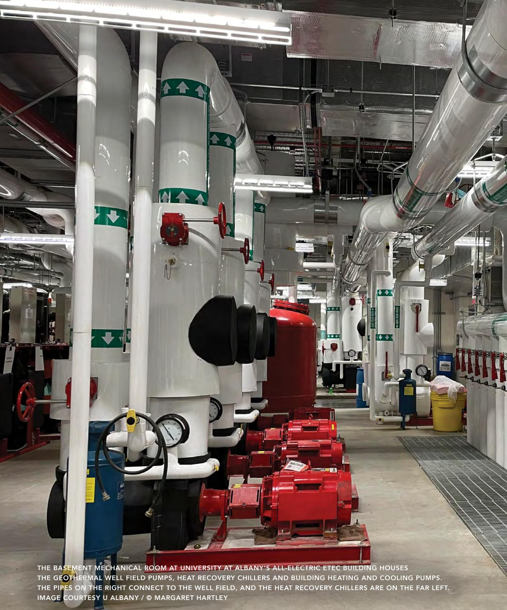
THE BASEMENT MECHANICAL ROOM AT UNIVERSITY AT ALBANY'S ALL-ELECTRIC ETEC BUILDING HOUSES THE GEOTHERMAL WELL FIELD PUMPS, HEAT RECOVERY CHILLERS AND BUILDING HEATING AND COOLING PUMPS. THE PIPES ON THE RIGHT CONNECT TO THE WELL FIELD, AND THE HEAT RECOVERY CHILLERS ARE ON THE FAR LEFT. IMAGE COURTESY U ALBANY / © MARGARET HARTLEY
